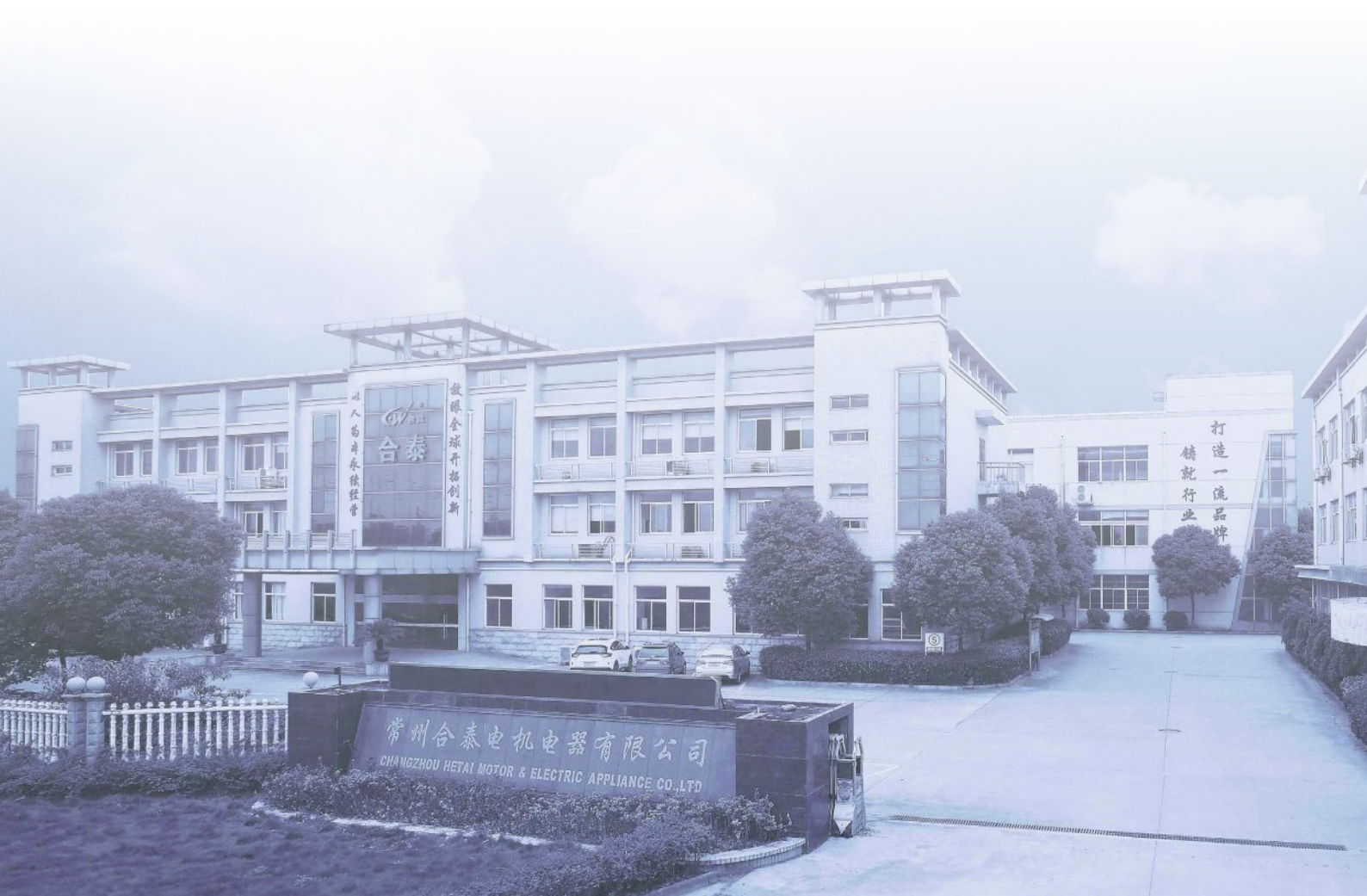
CHANGZHOU HETAI ELECTRIC MOTORS&APPLIANCE CO., LTD.
